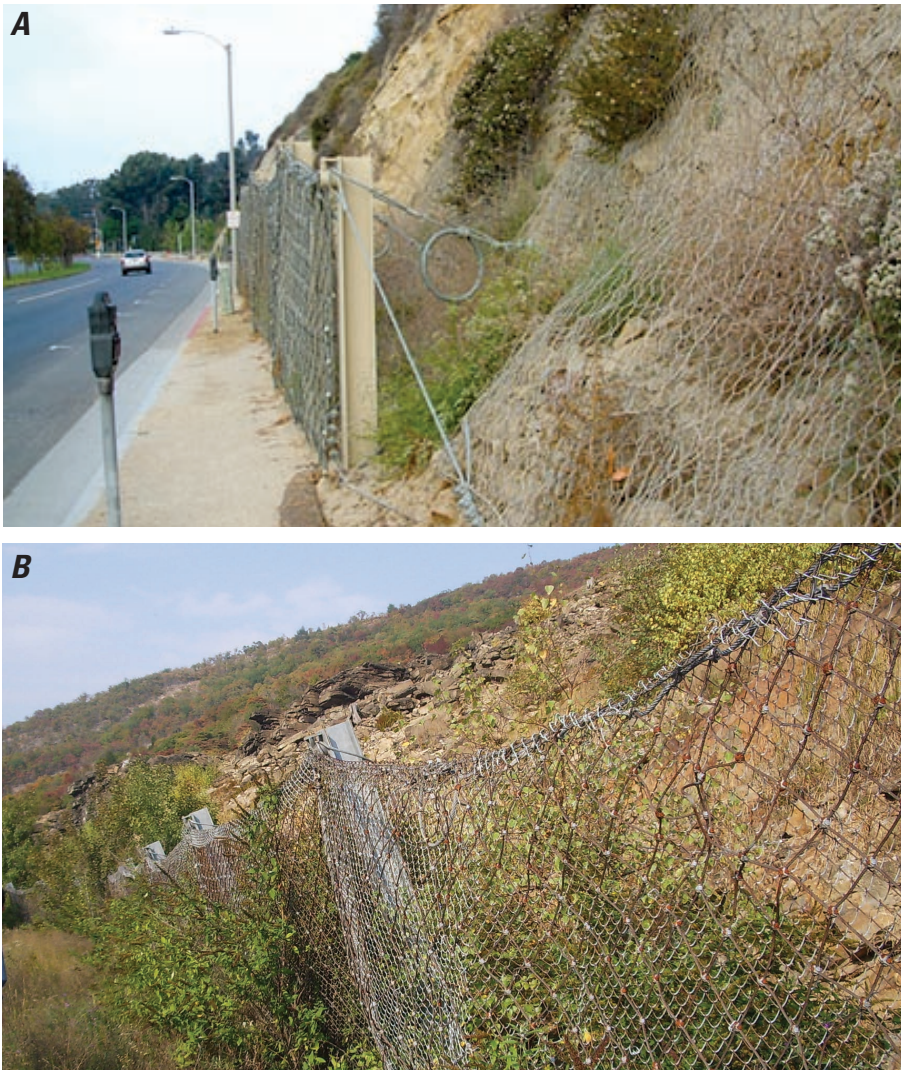
Figure C22. Protective rock barrier fencing along (A) a dirt trail in Pennsylvania, USA, and (B) a roadway in coastal California, USA. (Trail photograph, Lynn Highland, U.S. Geological Survey; roadway photograph from Federal Highway Administration, USA.)
